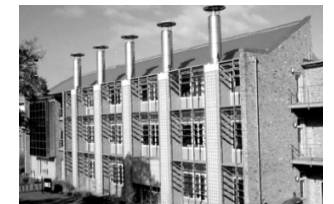
Motorised glazed louvers in the Environmental Office of the Future in Watford, UK
