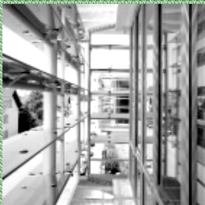
Glass lift/re system Gartner Design offices Gundelfingen Source: Gartner & Co
