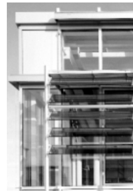
Glass louvre system Gartner Design offices Gundelfingen Source: Gartner & Co
