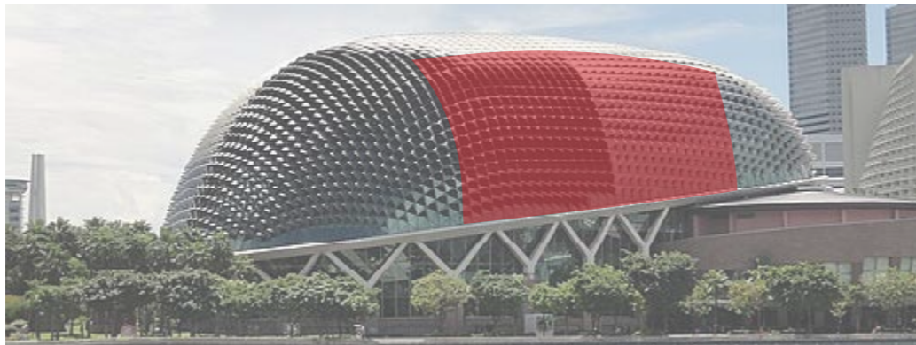
Figure 124. Esplanade facade used for case study.
