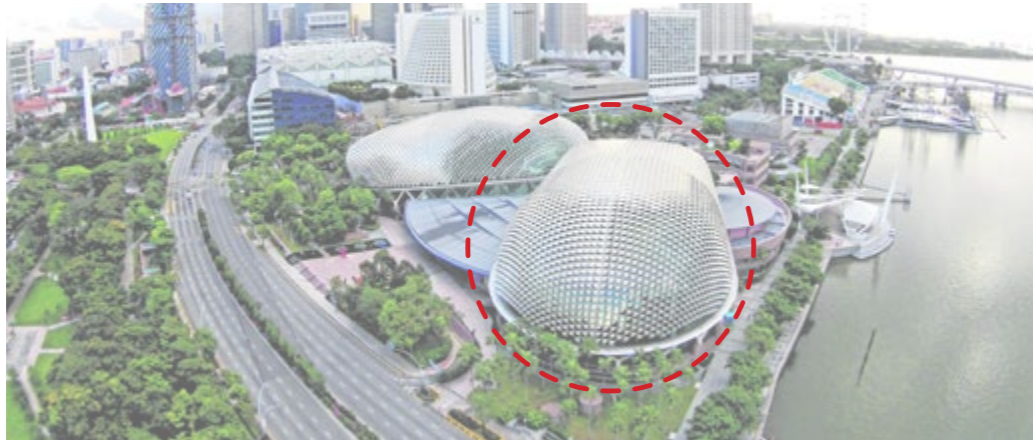
Figure 123. View of the Esplanade complex.
