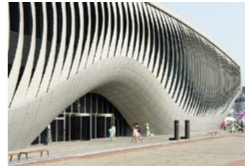
Figure 79. Bent and modulated metallic louvers
