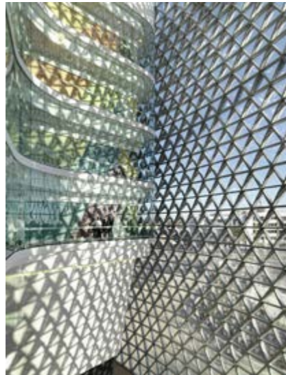
Figure 8. Building by Woods Bagot in South Australia, is an example of the use of static shading devices for indoor thermal comfort in large scale.
