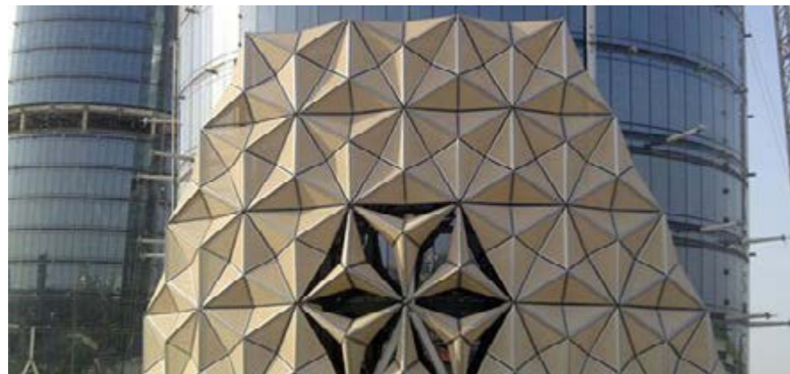
Figure 9. Al Bahar Towers in Abu Dhabi depict the use of adaptive shading façades with hi end technology, protecting a glass building in regions where high temperatures predominate.
