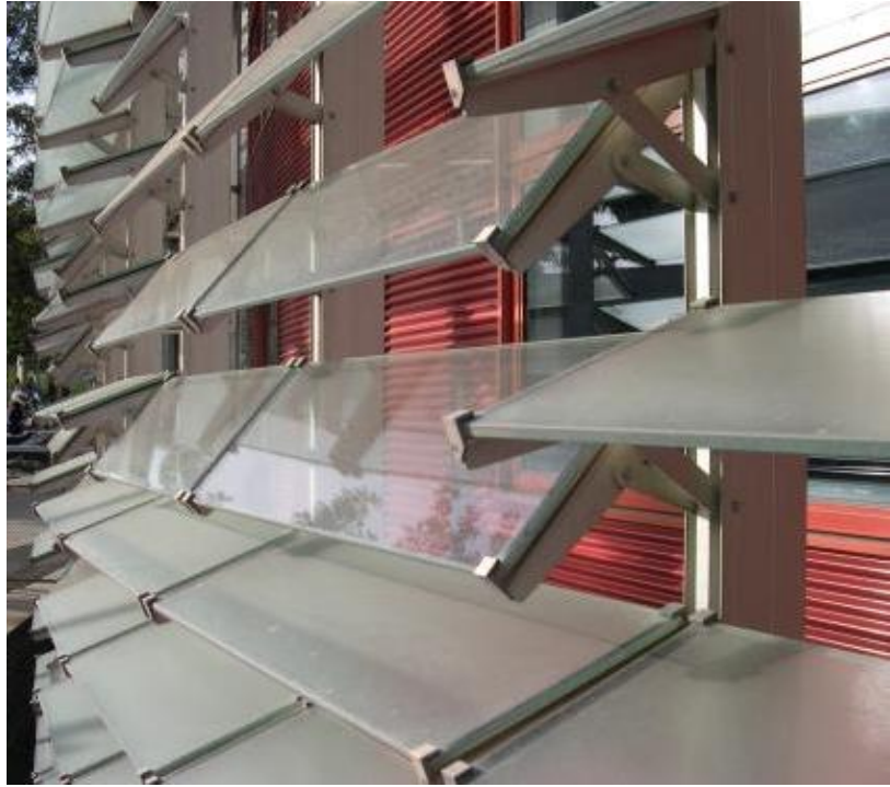
Figure 1-8: Detail of pivoting blinds (Web A-04)
