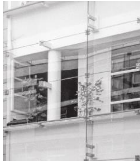
Figure 3-10: Principle box-window façade (side view) (Web 3-07) Figure 3-11: Example of a box-window façade (Klein, 2013)
