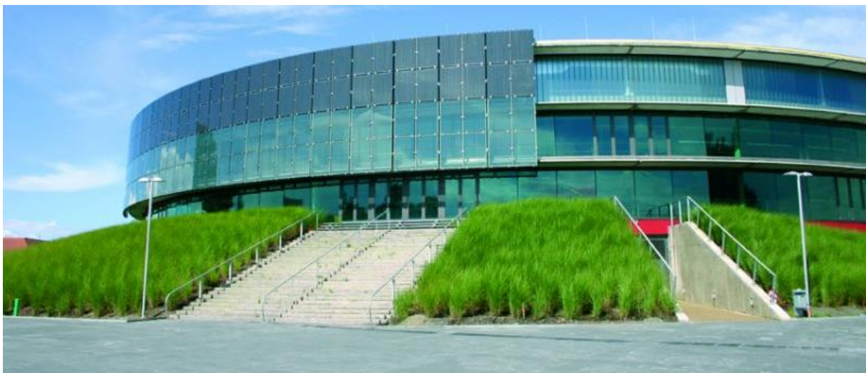
Figure 1-13: Controllable solar shading (Web A-07)
