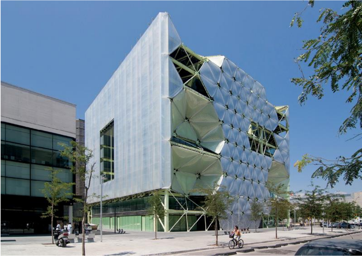
Figure 1-27: Media ICT-building (Web A-22)
