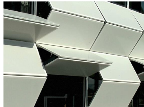
Figure 1-15: Detail of the façade (Web A-11)
