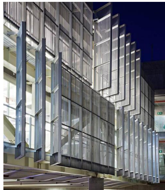
Figure 1-26: Brise-soleil cladding (from outside) (Web A-21)
