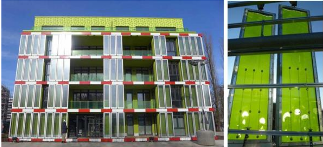
Figure 1-56: Solarleaf façade: a) front view, b) detail of two panels (Colt et al., 2013)
