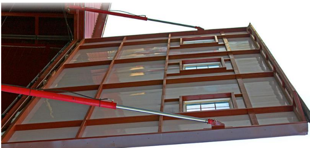
Figure 6-15: Hydraulic opening principle (Web 6-10)
