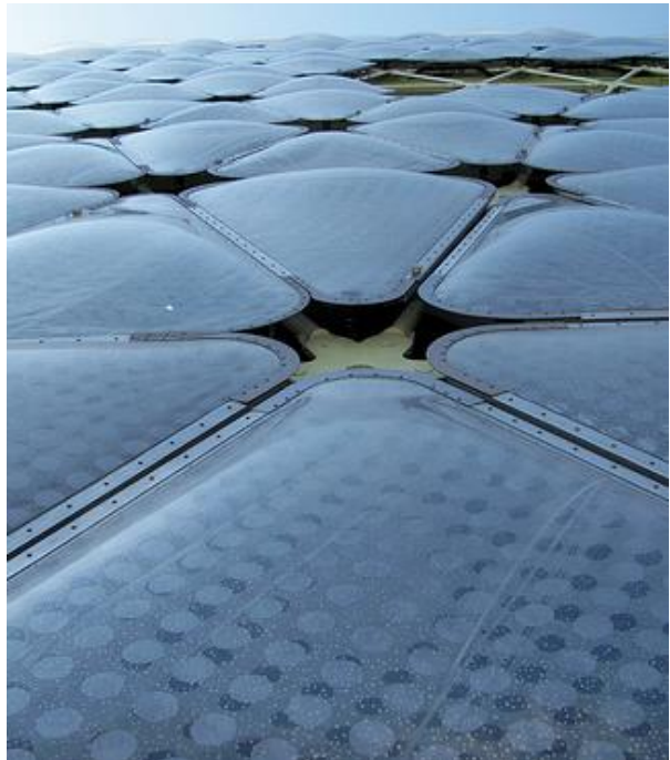
Figure 1-29: Detail of the inflating cushions (Web A-22)
